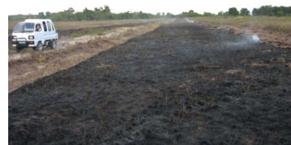
East view. Note grass burned in preparation for topsoil removal.
