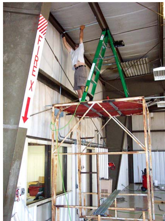
(Clockwise from the top left) Jim Holdeman and Andy Klein prepare the hangar floor for epoxy coating; The hangar before improvements; Mike Peterson from Randall Electric in Berrien Springs, MI installs conduit for new power wiring; the shiny new epoxy floor reflects light as the wainscot siding is installed.
