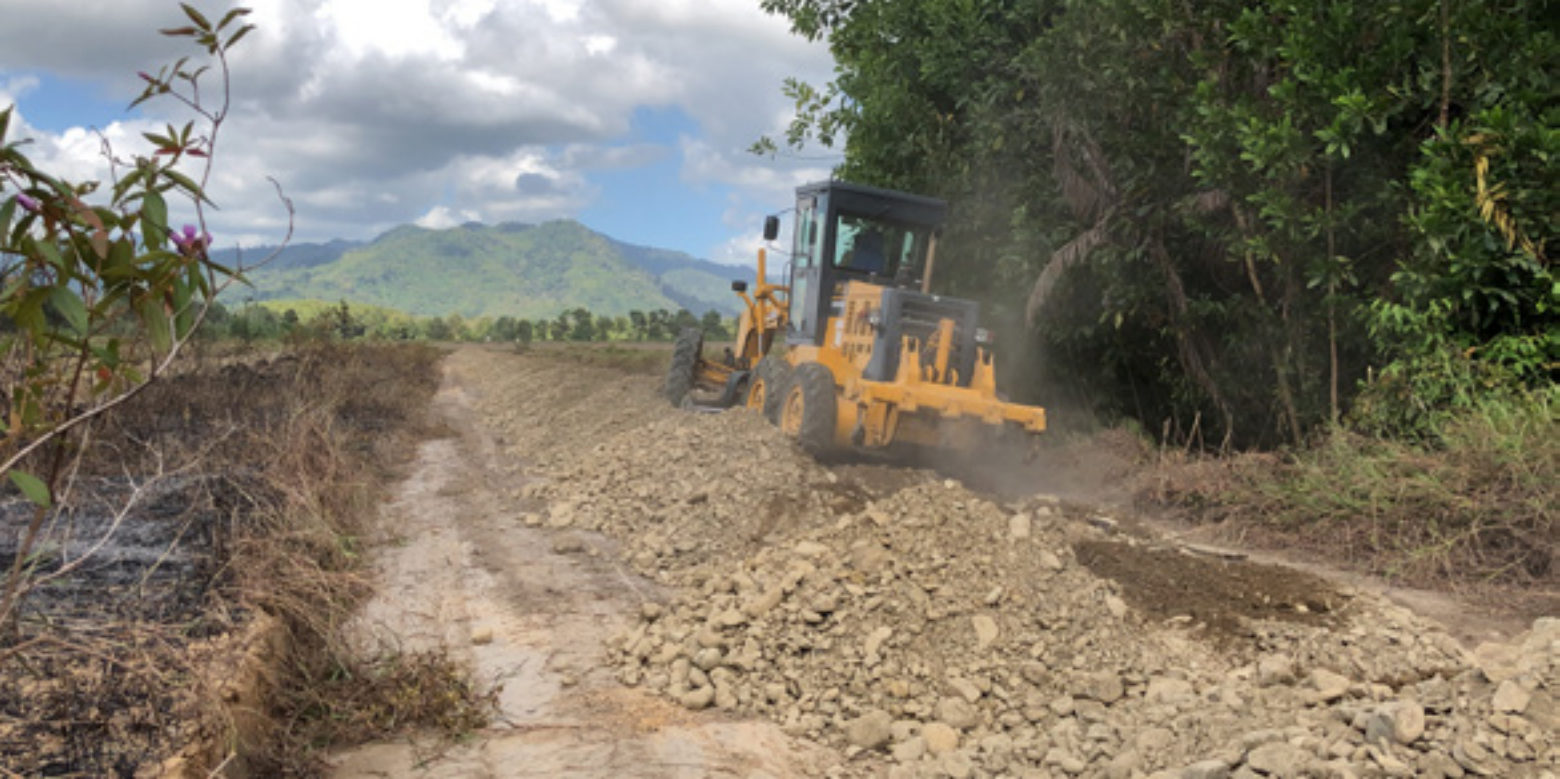
Grading the access road in the Philippines
