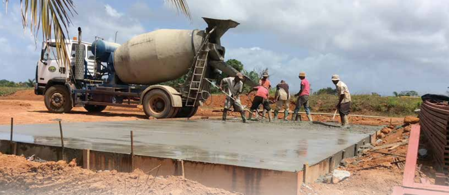
Cement finishing team carefully trowels the final section of the hangar floor.
