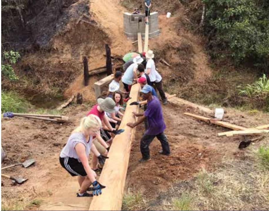
It took the efforts of nearly 20 people on the Nicaraguan mission team to maneuver the 1,500-pound beams that were used to construct a footbridge that enabled a local village to gain access for hunting, fishing, and farming.
